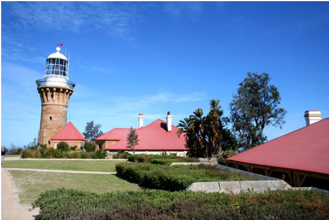
Photo 3 Barrenjoey Lighthouse heritage buildings. Michele Cooper/DCCEEW
