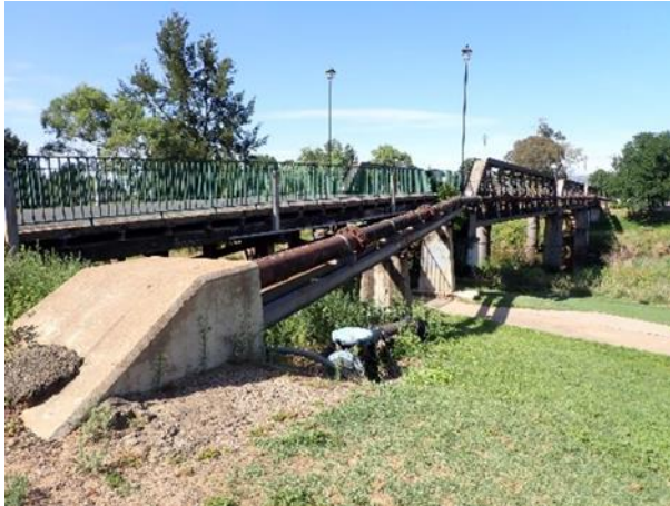
Figure 15 – East Service Pipes (Upstream)
