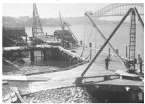
Figure 2.18 Reconstruction of the eastern wharf. Comparison with the above photo clearly shows that this wharf was completely rebuilt at this time. May 1944. SLNSW GPO1-07894.
