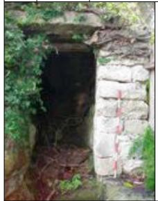
At the rear of the kitchen is an alcove partially cut into the rock face on the western side and constructed of 8 courses of stone on the eastern side. The roof consists of at least 4 large lintel stones 150 mm thick x 1250 mm wide x 680 mm long. The interior has been painted or lined in the past and measures 2.4 m in depth x 1.9m in height. This may have acted as a food or wood store although it is particularly well constructed and in good condition.
