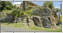
The north-eastern edge of the island was originally in natural form but was gradually reclaimed and reworked from 1901. The rock faces appear to be quarried to "square-up" the end of the island related to reclamation works. A dry stone retaining wall is constructed directly above to provide a small grassed area in front of the water police building.
