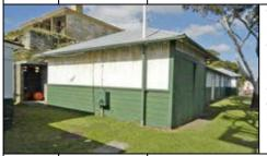
The Gear Shed replaced the earlier workshop building that was built to the shoreline. Built as part of the wharf upgrade and enlarged at each end around 1945-46 and following the relocation of the workshops to the shipyard precinct it is a lightweight building of timber framing with AC sheet and timber cladding with a hipped corrugated iron roof and multiple pairs of doors opening onto the wharf area, some with rail tracks to move heavy equipment. It is likely to have been reclad when altered.
