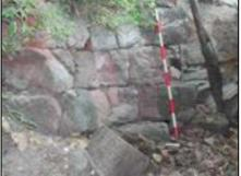
In the rock face to the rear of the boatshed the partial remains of a circular stone structure consisting of 9 courses of ashlar stone 2.5m high which would have had a diameter of approximately 1.5m. The retaining wall to the north on which the fig tree is growing was constructed later and on a different alignment to the circular structure. The construction of the retaining wall or the boat shed may have resulted in the disassembly of the structure and incorporation of the stone elsewhere.
