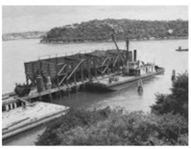
Figure 2.19 "Samson" Coaling. 9.1.1952. This is the clearest illustration of the coal platform that has now been removed. Also note the dolphins that were replaced when the new slipway was constructed. SLNSW GPO1-10051.
