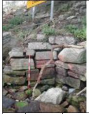
Located on the water's edge to the south of the kitchen and outbuildings. Consists of two stone walls 7 courses high (approx 1.2m) which meet at right angles at the base of the retaining wall and adjacent to the submarine cable. Large pieces of slate and numerous artifacts are located here as well. No documented evidence for its function.
