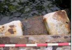
Wharf constructed of stone blocks partially visible extending from under the partially demolished timber wharf (55b). This area has been filled but originally served as the water police wharf from 1836.
