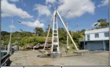
A 1940s jib crane mounted on the 1945 wharf with stiff legs on a concrete base. The crane is typical of small cranes from the period.
