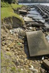
The eastern shoreline behind the eastern wharf has been progressively filled with building materials and debris probably for the last 90+ years. Unlike the northern wharves sea walls were not used to contain material. The shoreline is severely eroding and will in time return to the original rock shoreline.
