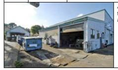
A simple skillion addition to the main workshop building of timber framing clad in corrugated iron. It has roller doors and was sited to avoid the rail system which closely abuts it.
