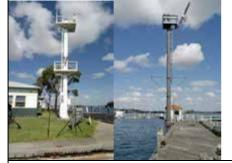
Front and rear tanker leads for tankers entering Gore Cove (day and night). One is on the ferry wharf and one on the corner of the filled area of the island. They replace earlier markers in similar locations. Date known from an MSB plan.
