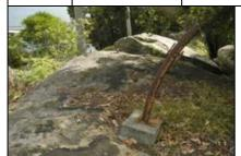
The signal mast set in a prominent location with clear views down the harbour comprised a steel post, now cut down, two sets of three guy points for signal ropes and four corner fixing points for stays. All of the fixings remain.
