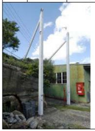
The fire brigade gallows remains only in part, missing its cross rails and braces. Used to hang drying hoses it also had pulleys and ropes. It was an essential part of the fire brigade infrastructure. It was braced back to the rock face and was adjacent to a timber access stiar.
