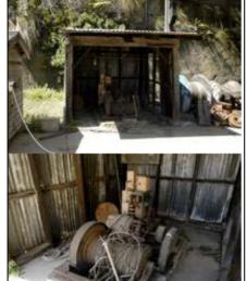
A simple timber framed corrugated iron clad skillion roofed shed located immediately north of the Scow Shed (16), housing the winch mechanism that powered the rope line, moving vehicles on the rail tracks from the wharf up the gentle slope to the magazine area. While the tracks have been removed or covered over, the winch and its housing and shed remain.
