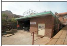
A utilitarian brick shed with open section housing the winch and a secure area housing the winch motor. The shed has a flat roof. Built in conjunction with the 500 ton slip, it accommodates the winch mechanism.
