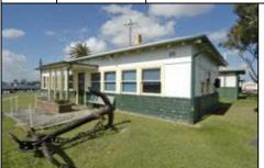
The dredge office is one of the last structures to be erected on this part of the island and had a specific use in relation to the operation of harbour dredges which were moored adjacent. it is of the same basic construction as the earlier Gear Shed with timber frame, timber floor, AC sheet and timber cladding and hipped corrugated iron roof. It has a small porch and has a better fitout than the other buildings in the area due to its office u se.
