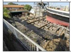
The 500 ton slipway required further excavation of the cliff edge and the magazine area to accommodate the rails, overhang and the winch house. This was the last major work to be undertaken in the shipyard.
