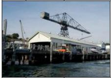
The first section of this shed to be built was the southern section with a floor level located at wharf height and apparently built over the earlier slip rails. Originally with central timber columns, they were removed and a steel support structure added to provide for clear spanning. A small mezzanine is located at the south end.
