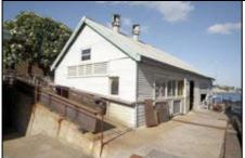
The corrugated iron clad and timber framed shed housing the winch mechanism for the 1949 slip and a stores area. It is gabled roof.
