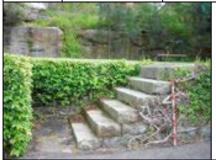
Same as 81b site of the former duplex constructed in 1913 is the most indicative of all the residential sites. The area has been terraced and a stone retaining wall faces the path on the northern side. Concrete stairs lead up to the building platform which retains the concrete front veranda and evidence of the wooden railing at the front.
