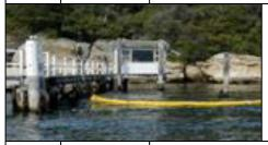
A small timber shed that has been relocated a number of times around the wharves and has had a range of uses. it is a basic and simple structure of timber framing and timber cladding.
