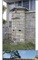
A coursed stone perimeter wall to the north, east and south of the magazine built on the edge of the quarry with a gateway, loop-holes and single sentry box on the southern alignment. The wall is finely dressed with even courses and the main gate is carefully detailed.
