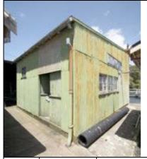
This building replaced a series of earlier buildings on the site also related to fire brigade use. It is timber framed clad with corrugated iron with a corrugated iron skillion roof. It is partially open with several secure rooms and appears to have built in several stages containing storage areas, secure stores, small workshops and later staff areas. It is a basic industrial structure with timber and steel framed windows, metal clad doors and fitout comprising workbenches.
