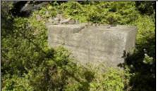
The mass concrete mounting blocks for the 1914 period crane set over the first wharf and quarry base. Only two of the three bases remain, one being removed for the Port Services Building construction. They have holding down bolts for the steel superstructure still in place.
