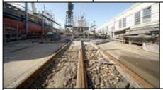
The 150 ton slipway retains its original formation near the water with the use of timber logs to support the rails and stone infill, the higher levels have been upgraded with concrete construction.
