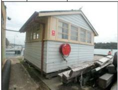
A movable building with an MSB number over the door indicating it was moved a number of times. It appears in several photos in different locations on the island. It is timber framed and clad with weatherboards with a gabled iron roof and windows to all sides.
