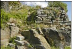
An early set of stone steps, probably dating from the time of construction of the water police station leading down to the point. The edge of the escarpment has been built up with dry stone walling to retain the upper level area in front of the building. The lower edge of the photo shows further excavation.
