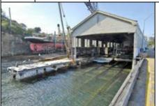
The first slipway to be constructed by the SHT remains adjacent to the broadside wharf and now partially covered by workshop buildings. Cut into the base rock along the shoreline it did not require excavation of the cliff face as the later slips required. It comprises 2 sets of iron rails fixed to the sloping rock base.
