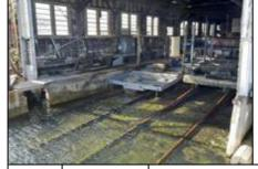
An addition to the workshop building that provided cover over the upper part of the 1926 slipway for working on vessels, this is the only covered section of slipway. It is a timber framed building with timber trusses with a perimeter walkway.
