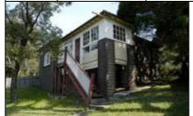
A Former Fire Brigade face brick cottage built 1922 to a different design to the earlier remaining cottages reflecting the change in styles from federation to interwar periods, with hipped roof and unglazed terracotta tile roof. The cottage is elevated on brick piers and has extensive views to the harbour to the east. The front verandah on the northeast end of the front (east) elevation has been enclosed. Windows are timber-framed multi-paned double-hung. The timber front steps are deteriorated.
