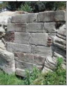
The lime kiln is located just to the east of Anderson's couch. It is cylindrical, overgrown and silted up, measuring 2 m diameter and is 2.2 m deep. While it is constructed partly of ashlar blocks and brick, much of the structure is cut into the natural contours of the rock outcrop. Slag is used in the mortar and the kiln contains associated ash and lime deposits and evidence of high temperature burning.
