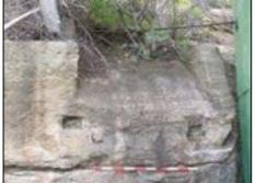
Remains of the stairs leading down from the Water police precinct to the wharf/jetty constructed in 1836 on the northern side of the Island. Photographic evidence shows the wooden hand rail and stairs still in place in 1945. Only 4 rectangular slots for rails now remain cut into the rock face and a cut 1m wide ramp where the wooden stairs were likely to be located.
