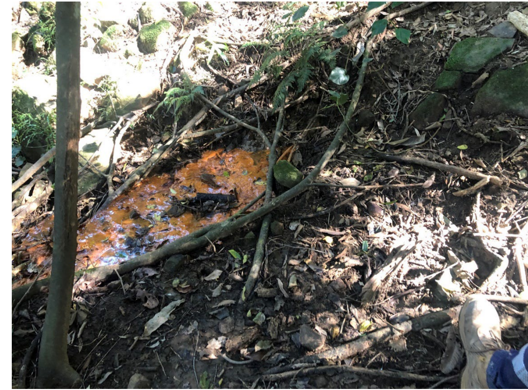
Terrain Unit 3 Photograph 2: Seepage along the level terrain along the toe of the steep bench slopes.
