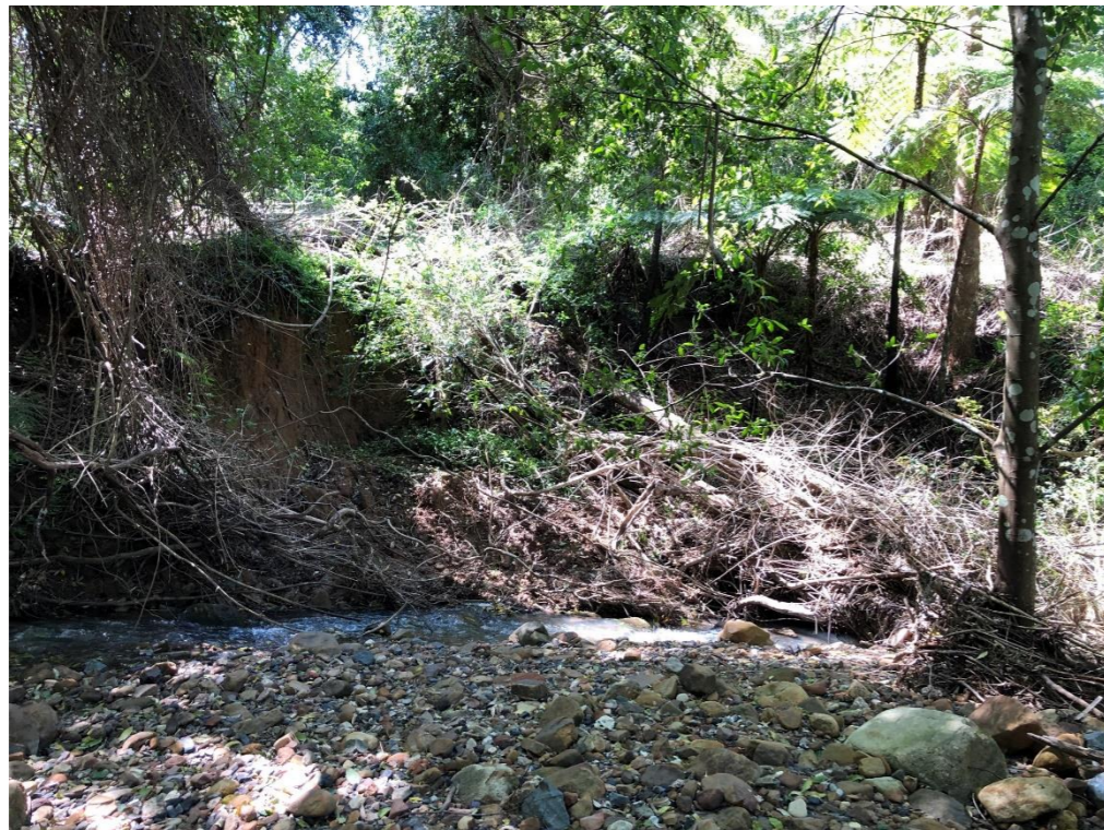
Terrain Unit 5 Photograph 5: Slumping along sections of the river.
