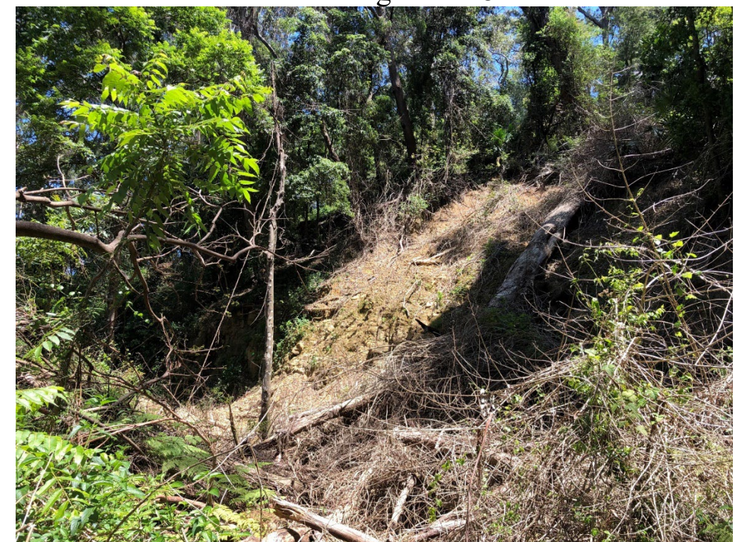
Terrain Unit 2 Photograph 24: View of overburden soil washout.
