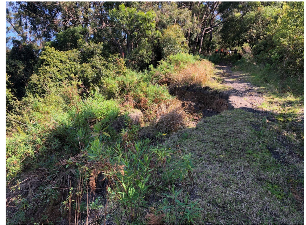
Terrain Unit 2 Photograph 8: View of slip along access road from the Corrimal Colliery.
