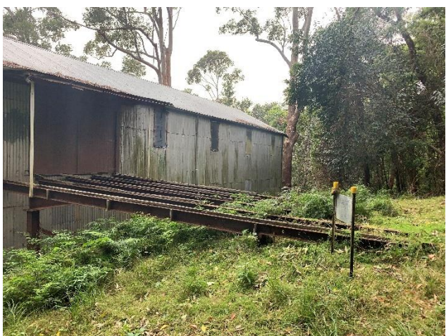
Plate 67: Ramp made of rail girders (Source: Niche)
