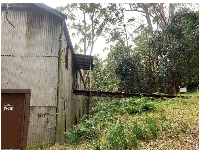
Plate 65: Ramp to first level of building (Source: Niche)
