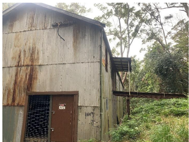
Plate 66: Outside of building (Source: Niche)
