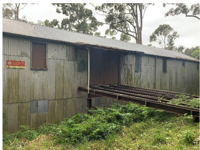
Plate 68: Ramp made of rail girders (Source: Niche)
