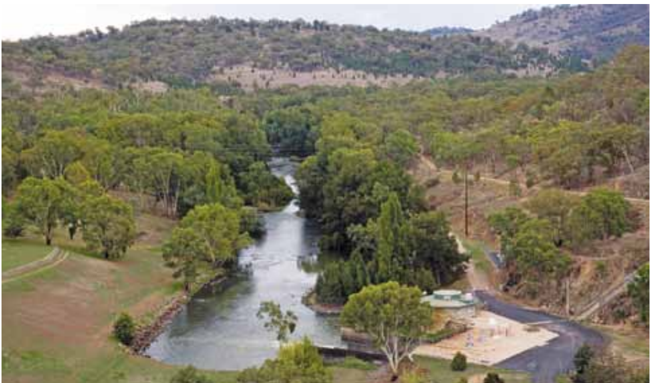
Photo 19 A view downstream at the Burrendong Dam outlet (Grenville Turner).
