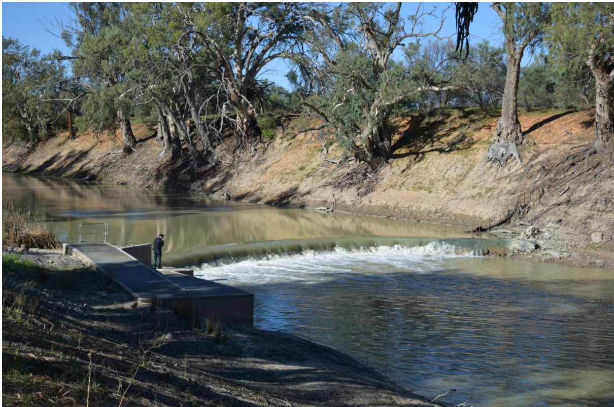
Figure 5 Burtundy Weir and fishway on the lower Darling River Photo: DPIE
