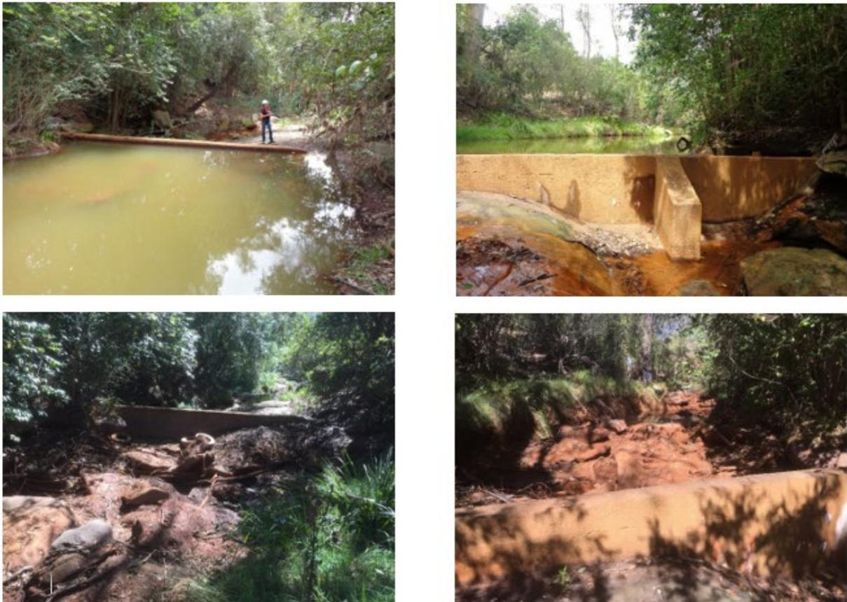
**Figure 3.8** Redbank Creek weir pool looking downstream (left) and looking upstream at the weir wall (right). Prior to LW31 impacts above (photos taken 24/2/17); after LW31 impact below (photos taken 28/3/18)
