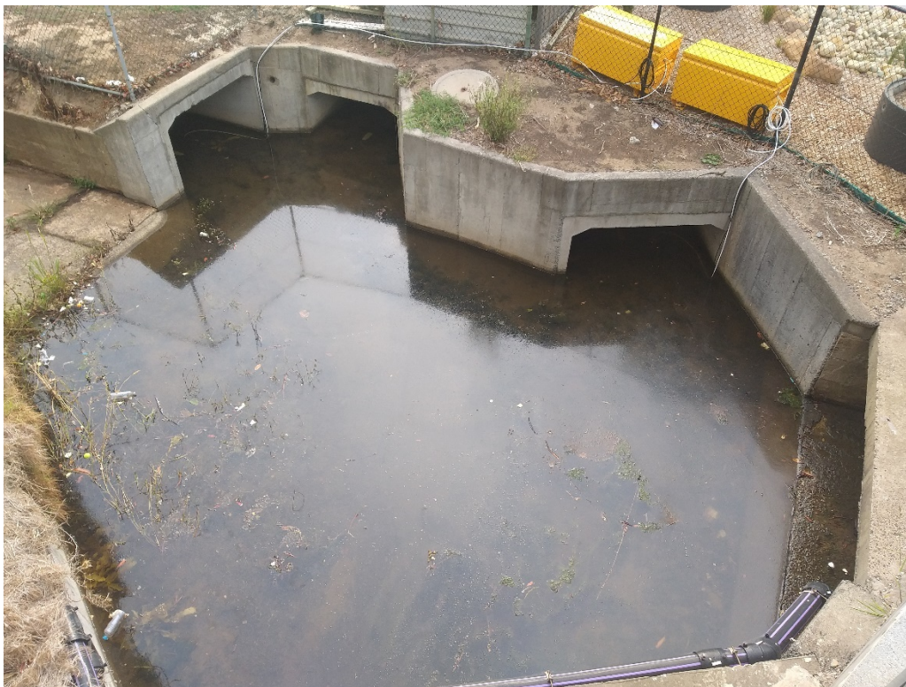
Autosamplers at Terrigal, upstream on seven drains. Photo: DPIE
